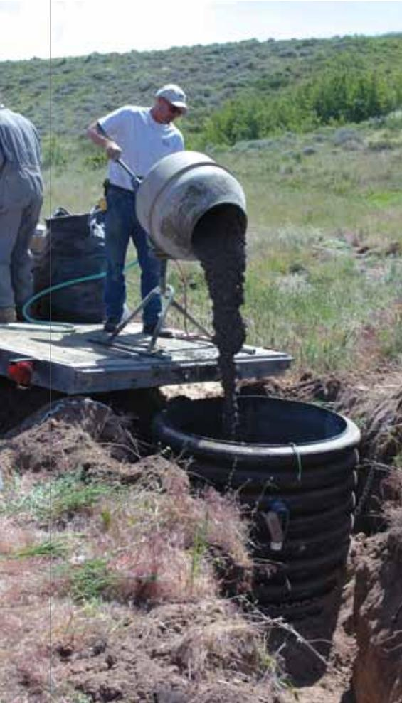
An EarthScope technician pours concrete for the base of the tank that encases the USArray seismometers.
