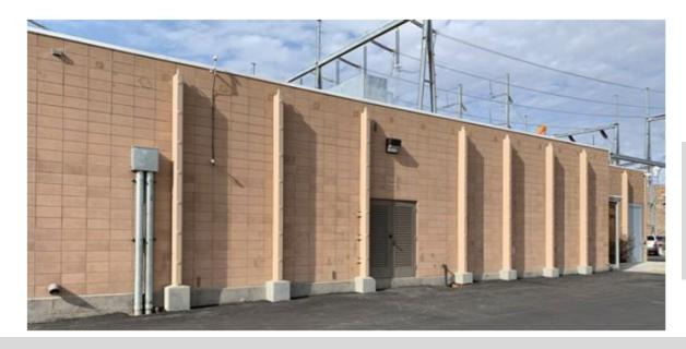
'Strongbacks' are pipes attached to an exterior wall of a MEER
