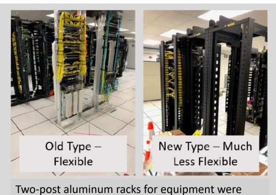
replaced with 4-post seismic qualified racks to
