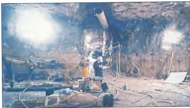
Figure 1. The explosive chamber, known as the "tuna can," which was filled with a blasting agent for NPE. The cavity was filled with nearly 1.3 million kg of the agent and produced a seismic signal which had a magnitude of 4.1. Photo courtesy of Jay Zucca, Lawrence Livermore National Laboratory.
